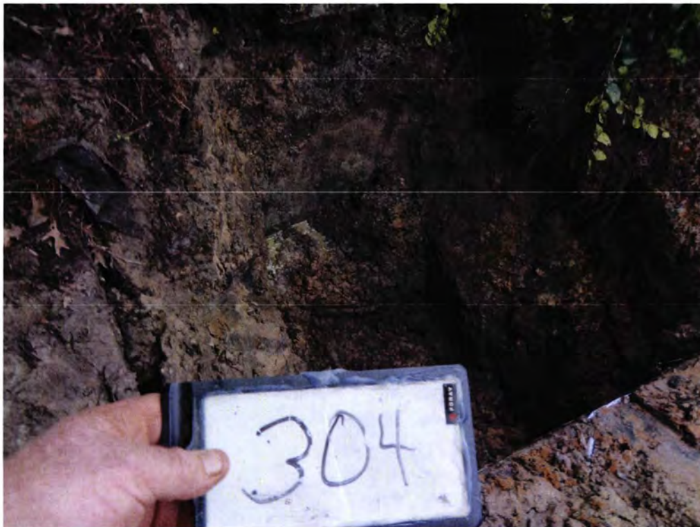
Picture 2: UST 304Ash excavation.
